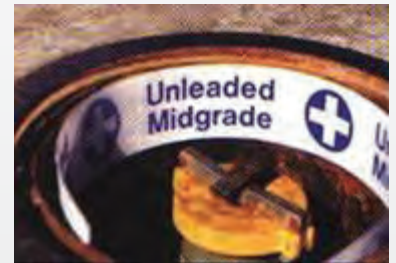
Installed Tank Collar >>
